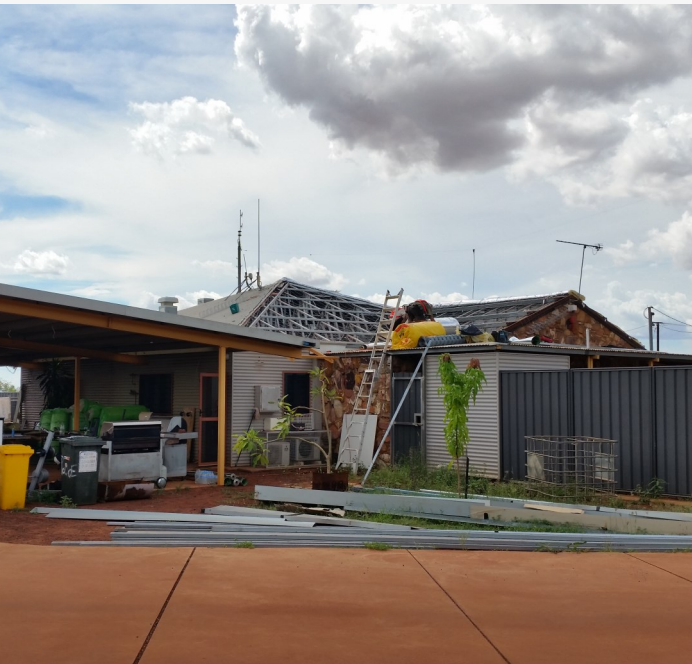
MGCBM refurbishment of the Balgo Police Station
