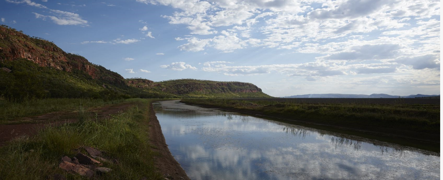
M2 Irrigation Channel
