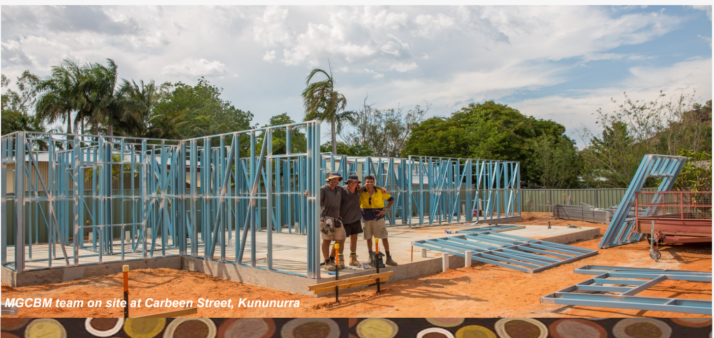
Residential development in Carbeen Street, Kununurra
