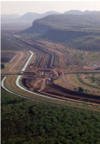
Work on the channel and road extension for Ord Stage 2
