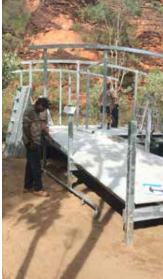
Eco-construction work at Mirima
