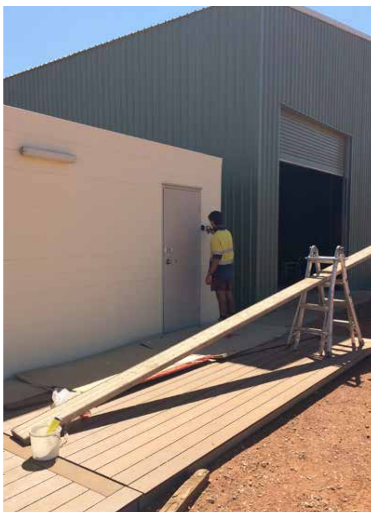
Kentia Way office block
