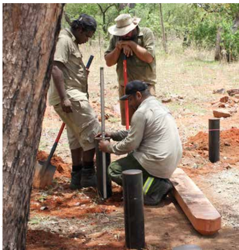
Wayne Winton and Winston Gerrard installing bollards at Black Rocks
