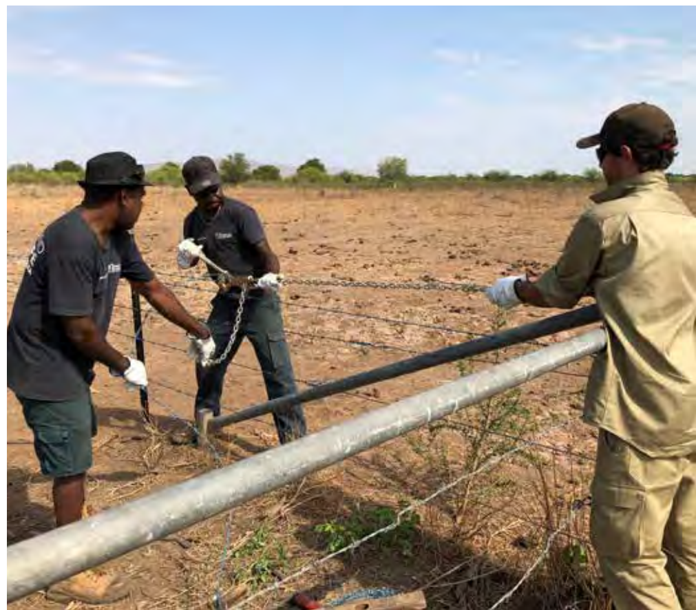
Fence construction at Carlton Hill
